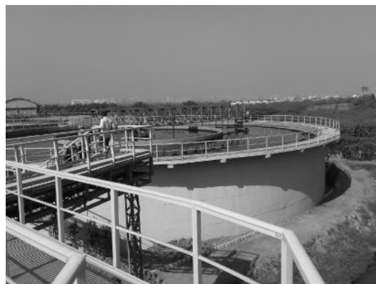
Site Visit at CETP Pandesara, Surat for CETP upgradation project
