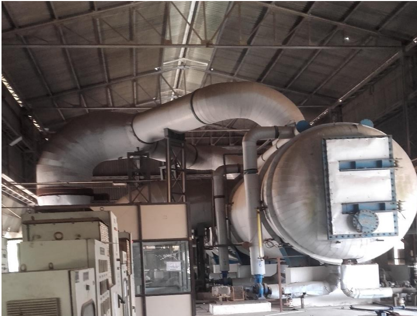
Mechanical Vapor Recompressor (MVR)
